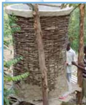
Water tank made from woven reeds and plastered inside
